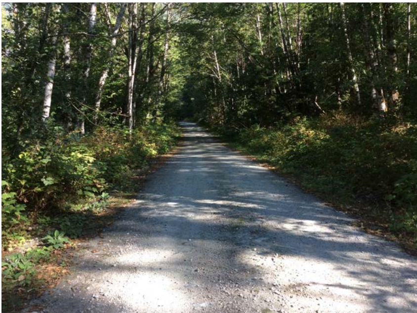
Right approach viewed from bridge
