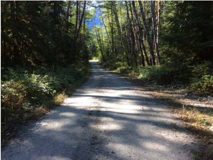
Left approach viewed from bridge
